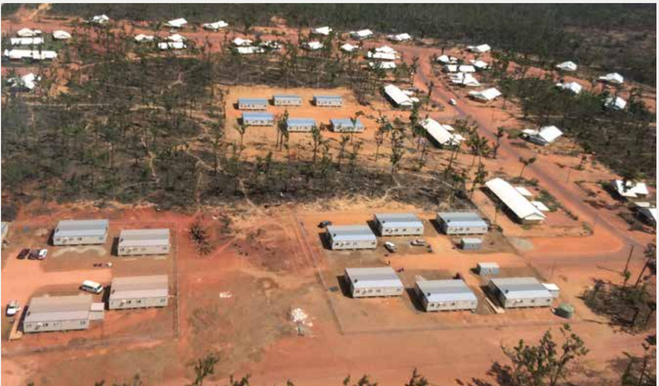
Galiwin'ku: three of the seven clusters of temporary housing mobilised and installed in Galiwin'ku as part of the $100 million cyclones Lam and Nathan rebuilding program. This is one of the largest logistics projects ever undertaken by the NT Government with more than 40 temporary houses mobilised via barge and installed.
