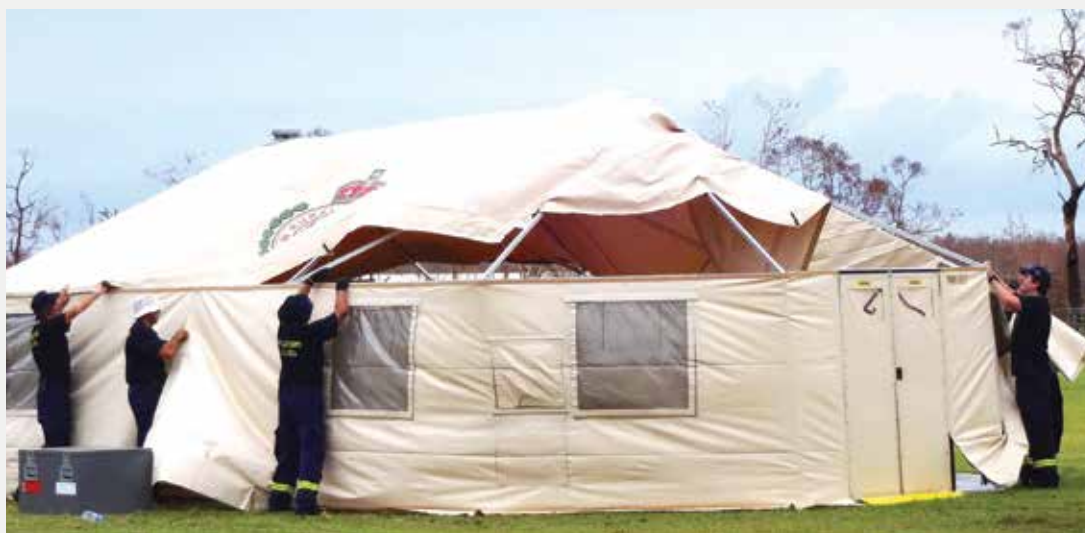
Galiwin'ku, Camp Elcho – shelter construction.
