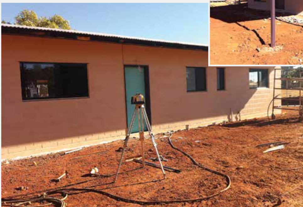
Tennant Creek, youth accommodation facility under construction.
